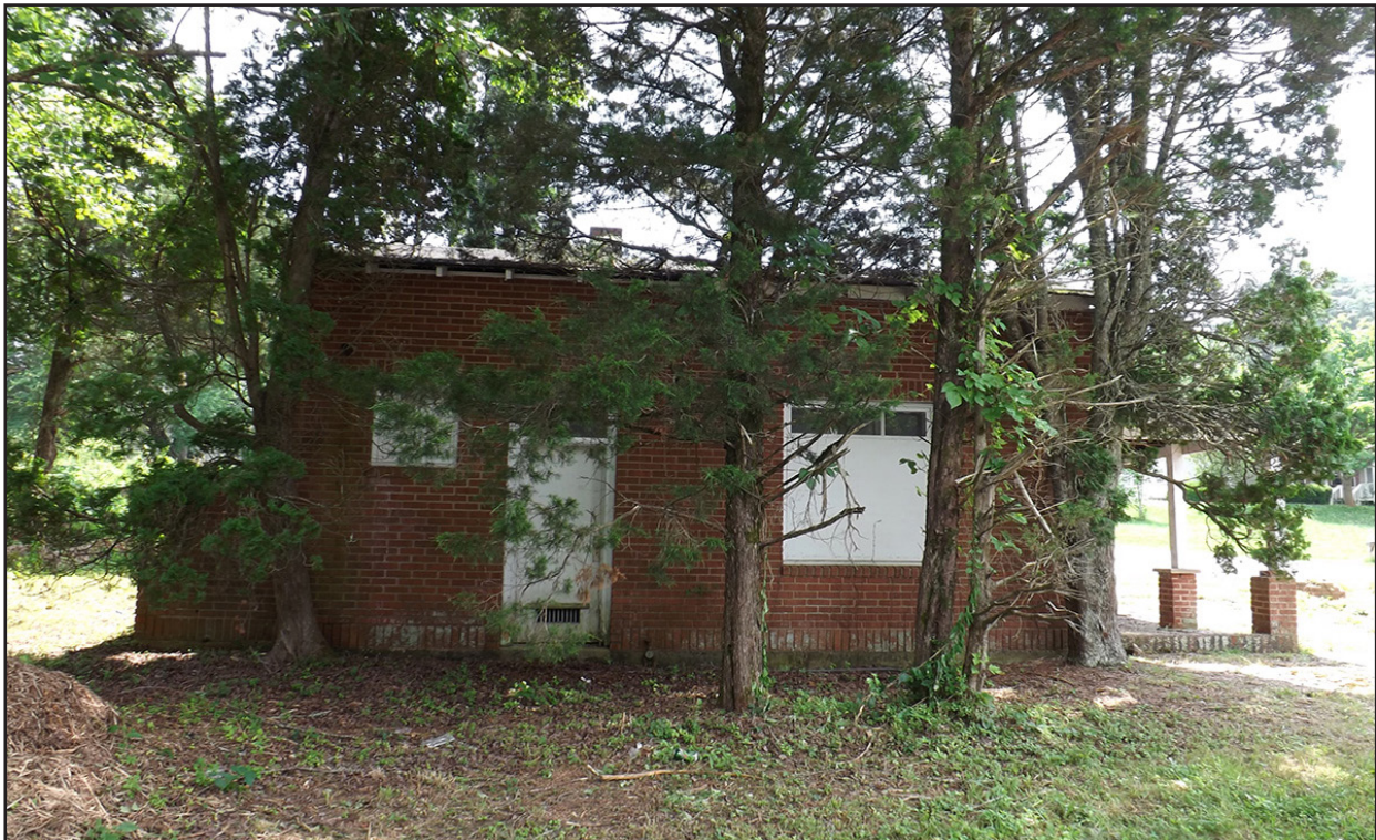
Figure 9. Property CY0036; view is south and features the north elevation of Chatuge Tavern.
