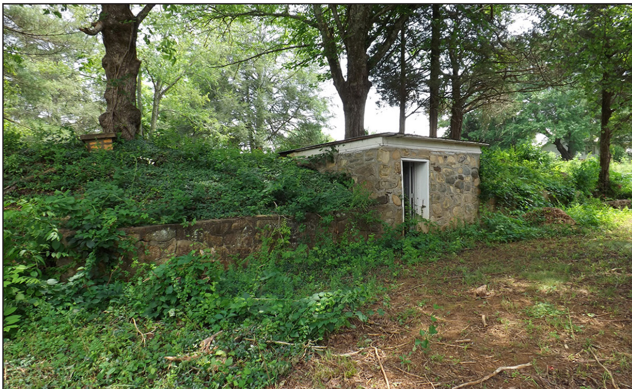
Figure 16. Property CY0036; view is southeast and features the bank cellar.
