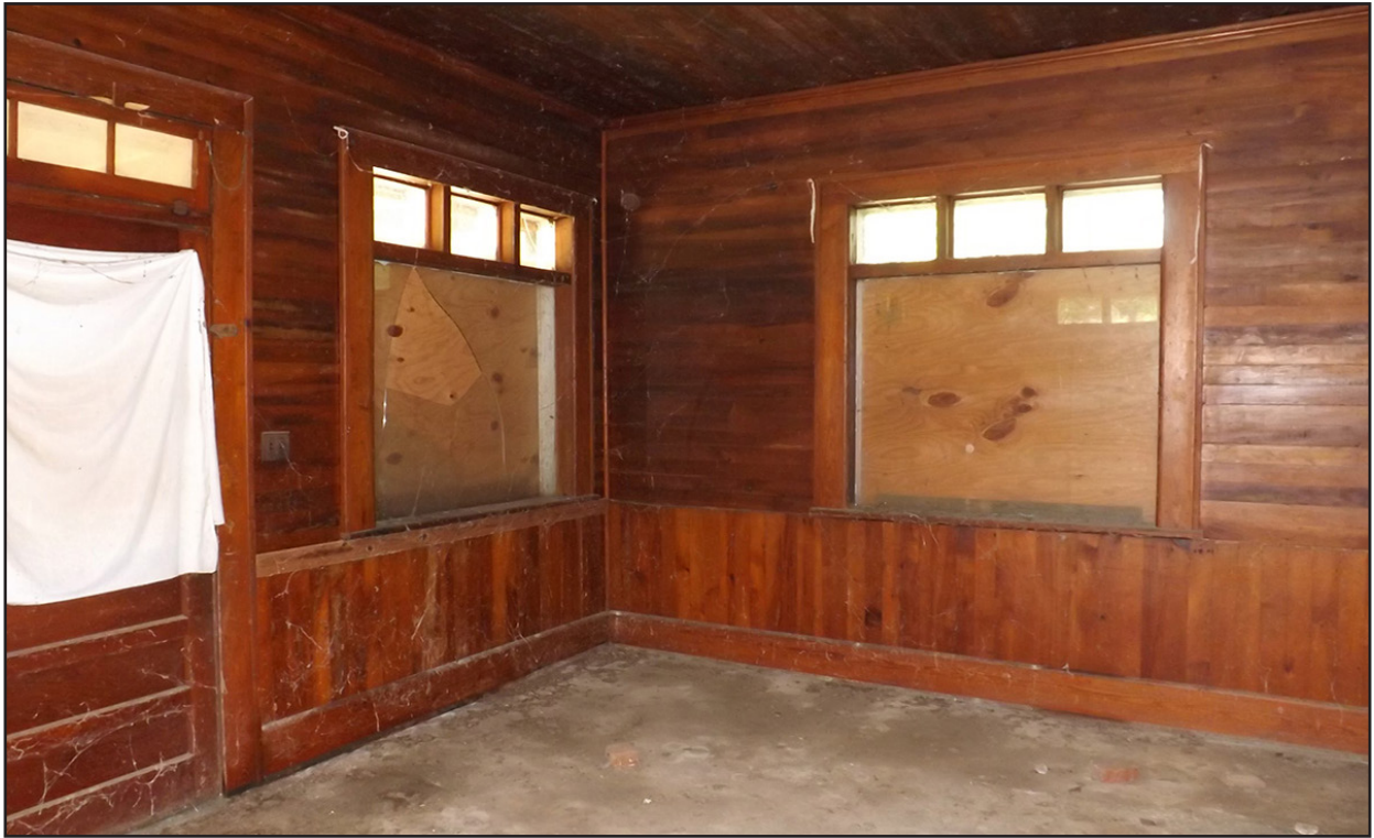
Figure 10. Property CY0036; interior main room of Chatuge Tavern; view is northwest.
