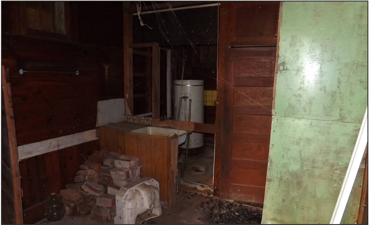
Figure 14. Property CY0036; interior of back room of Chatuge Tavern featuring the bathroom.
