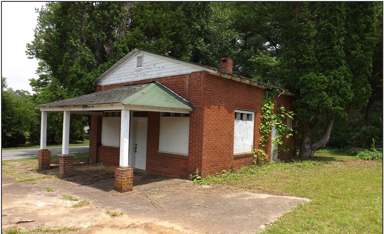
Figure 7. Property CY0036; view is northeast and features the façade and south elevation of Chatuge Tavern.
